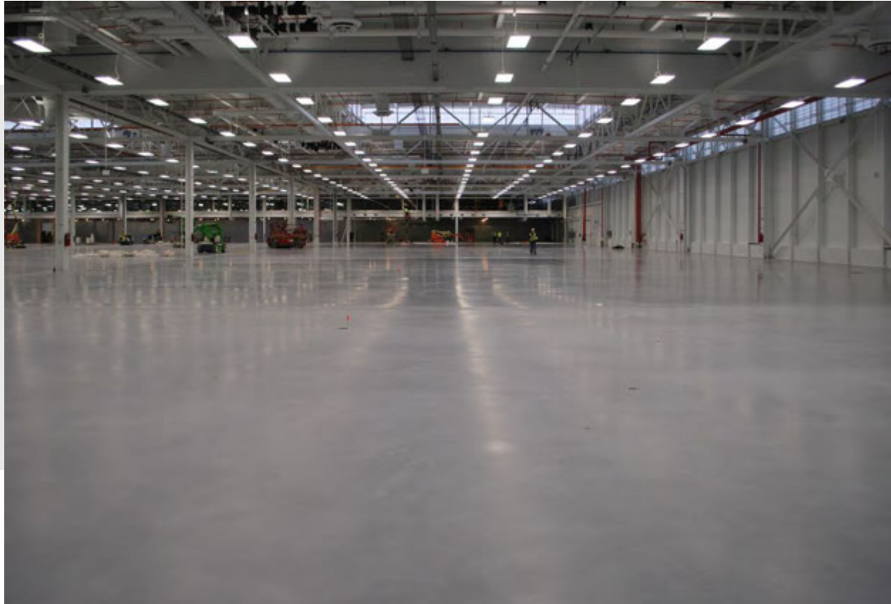
Joint-free concrete slabs on grade. Image courtesy George Garber
