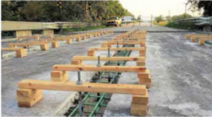
Fig. 2: Joints between reinforced concrete beams were replaced with UHPC. Dimension lumber portals and threaded rods held the bottom formwork tight against the beam flanges to prevent leakage of the UHPC
