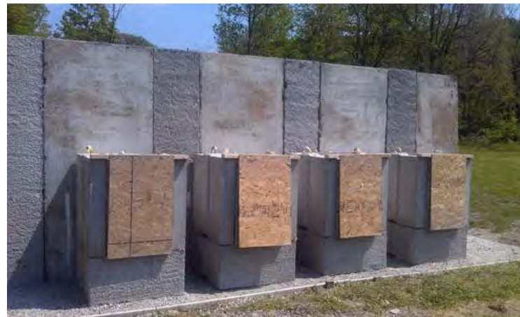
Shock-absorbing concrete, bullet traps
