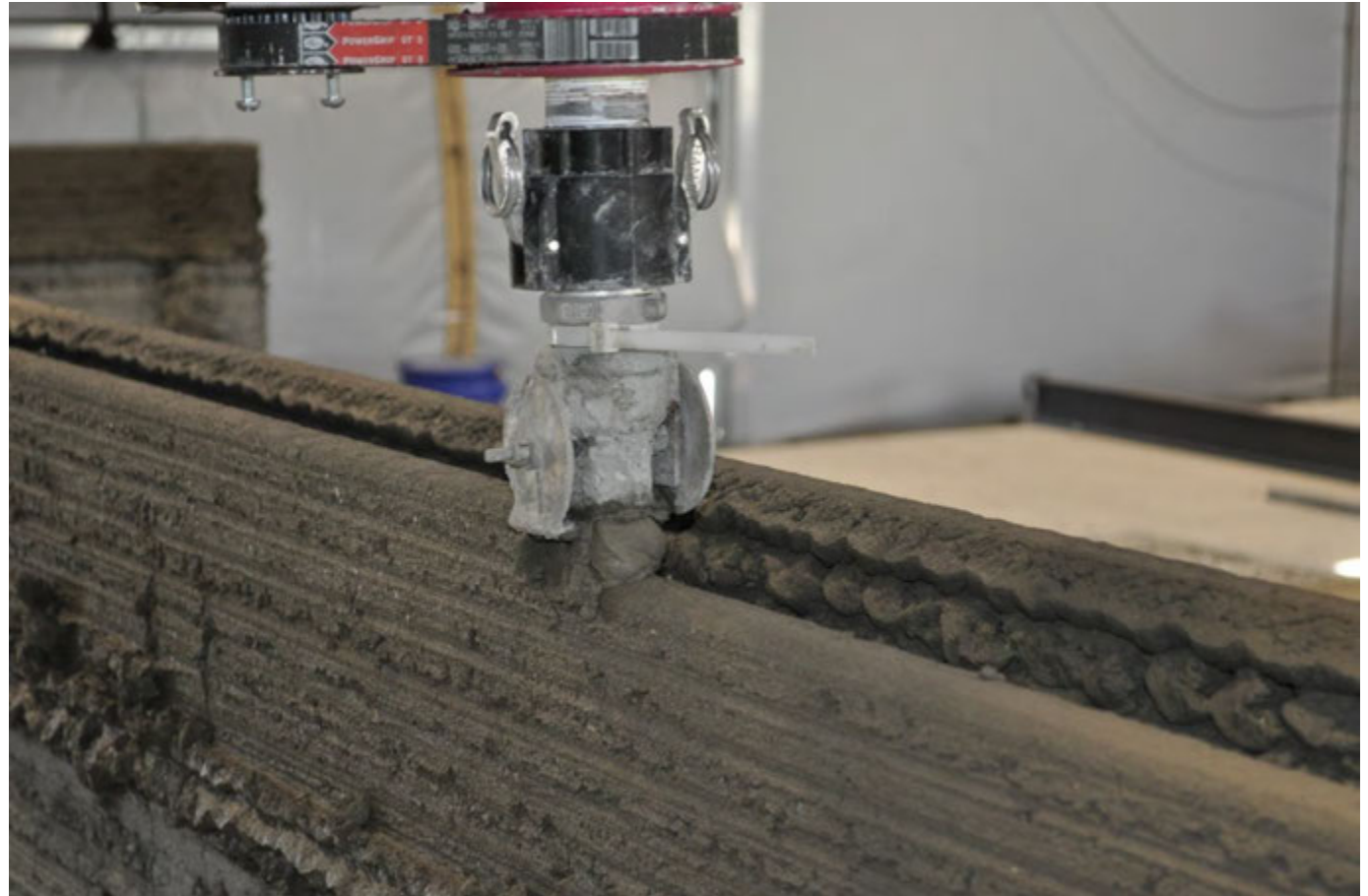
A printer head from the 3D printer ACES at CERL
