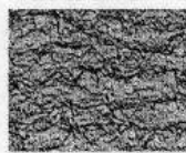
CSP 9 (heavy scarification)
